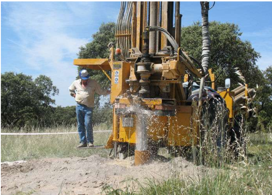
Spain ~ Naval Moral | Drilling on the top of the mountain. Contact with water at 42.5 M | Filling: approx. 15 m 3 /h
